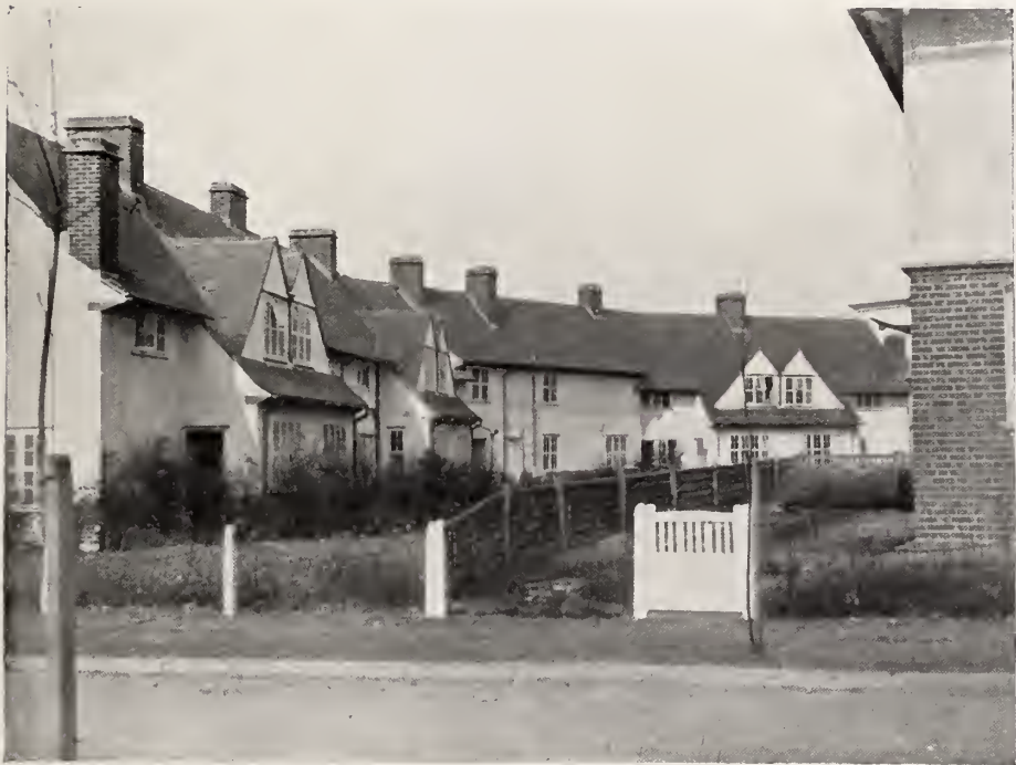
Illus. 239.—Hampstead Garden Suburb. View of the Backs of some of the Hampstead Tenants' Cottages. Contrast Illus. 237 and 238.
